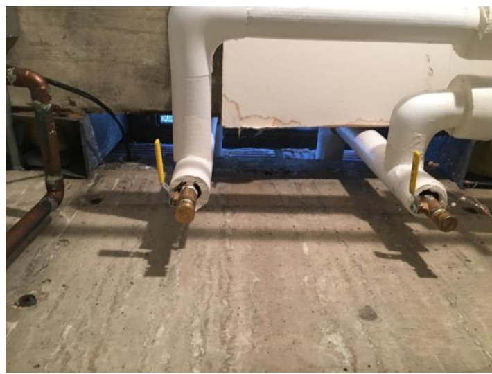
Top: Water staining at location of area well Bottom: Top of area wells below sidewalk
